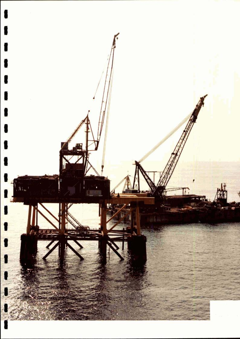
The support frame arrived on location and was set on the DP2 jacket on August 4 by the barge PM 27. The welding of the support frame/jacket connection was completed on August 10.
