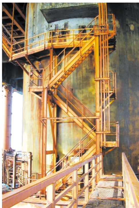
Figure 6.3 Stairways and Walkways Below Deck Level on CDP1
