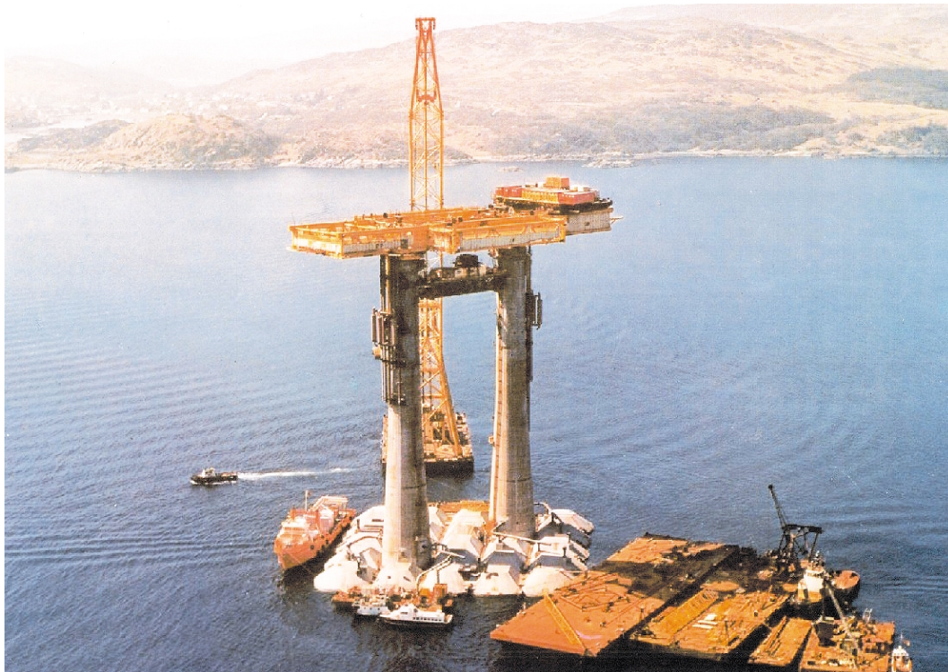
Figure 5.11 Construction of TP1 after Installation of the Deck Structure
