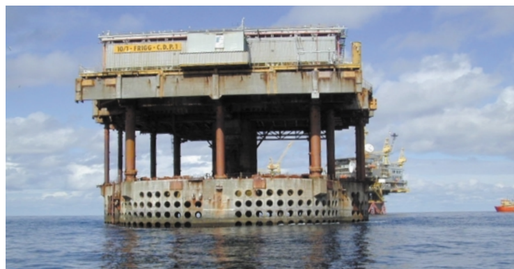
Figure 5.6 Present Condition of CDP1
