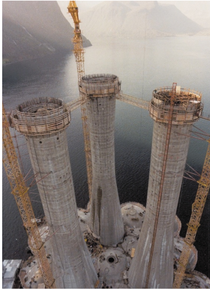
Figure 5.5 TCP2 During Construction
