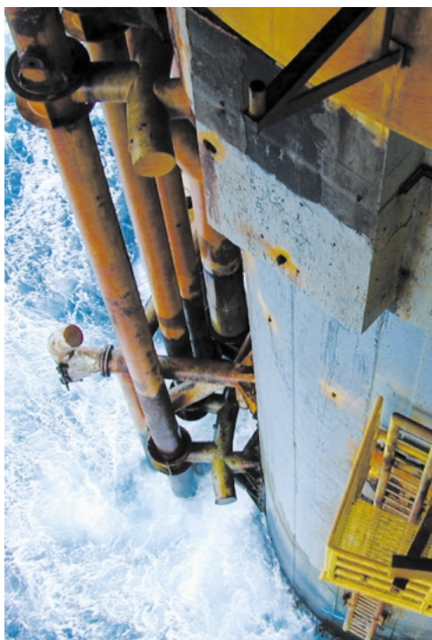
Figure 6.2 Risers and External Steelwork on the Outside of TP1 Column
