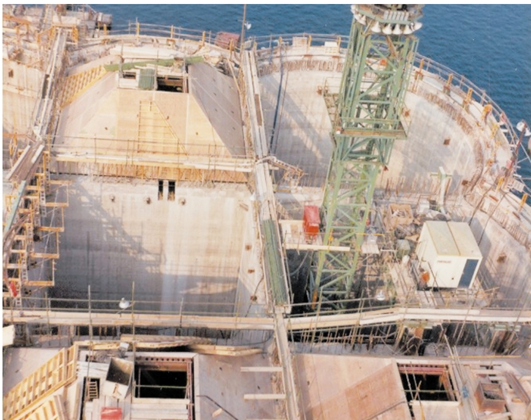
Figure 5.14 Construction of the TP1 Substructure showing the Internal Walls and Cells
