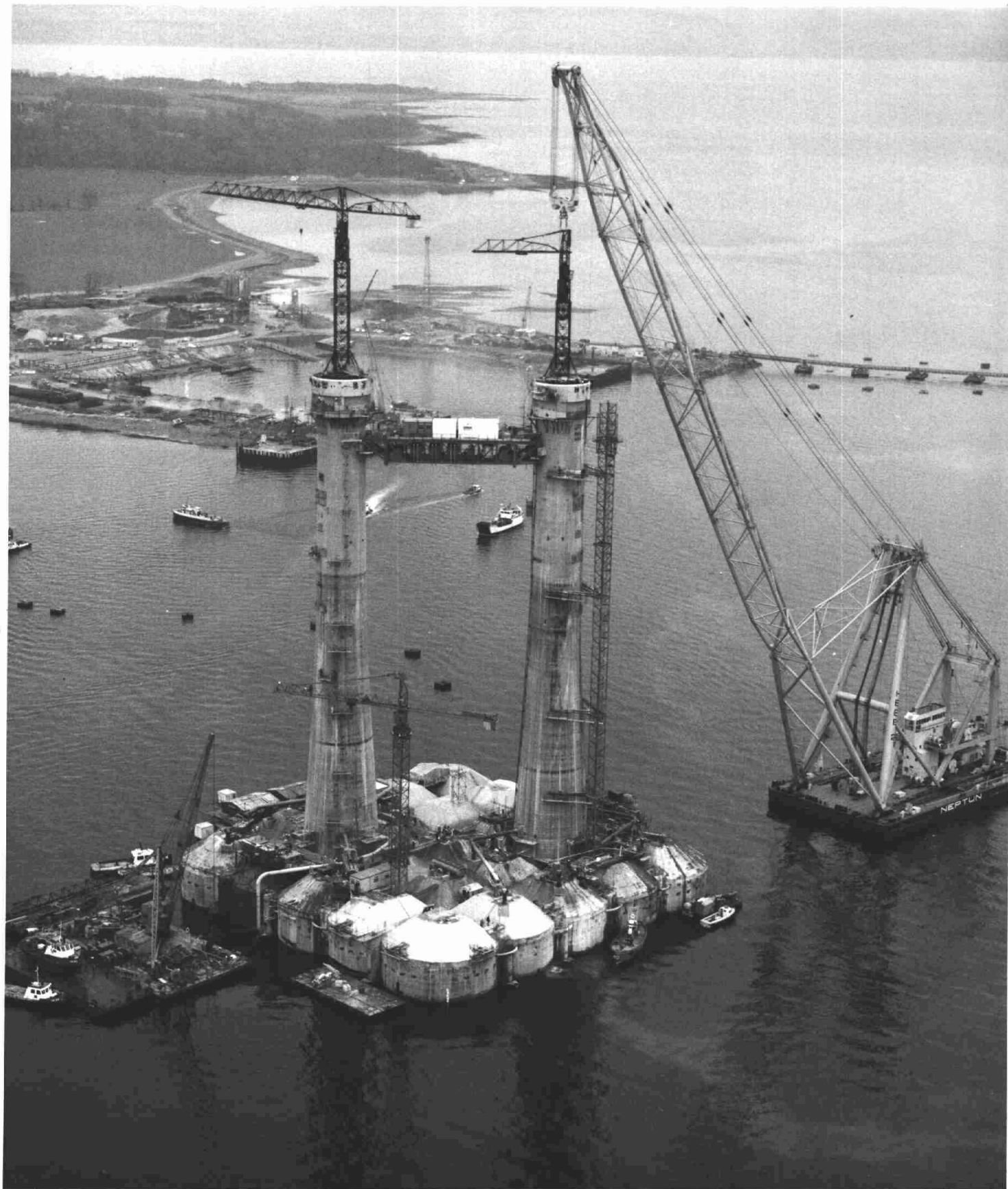
76/149/6 VIEW OF ELF T.P. 1. PLATFORM FROM WEST SHOWING 27.2.76. ERECTION OF TOWER CRANE TO COLUMN C. 1 IN PROGRESS.
