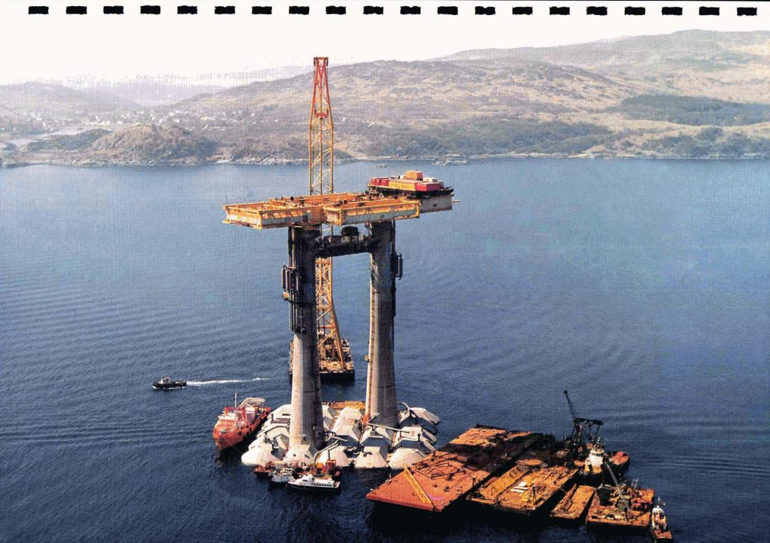
Pumphouse PH is complete. Load-out on the KARMOY occurred on May 24, 1976. Sea fastening is in progress.
