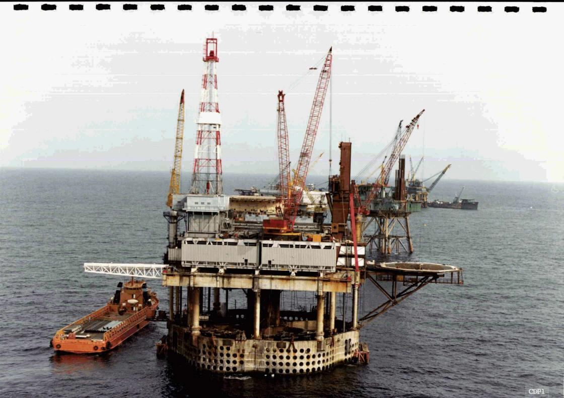
The south-west leg beam was offloaded on August 30. Dismantling of the north-west column was completed on September 8. The south section of the running beam and a northern brace were offloaded on the 16th and at the present time the Buzichelli gantry crane has been completely dismantled.
