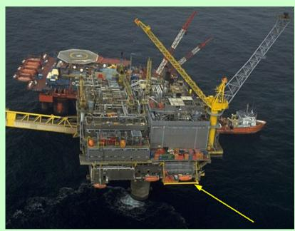
The module is also equipped with a pedestal crane at the SE corner of the module. The crane has the following working radius and SWL:
